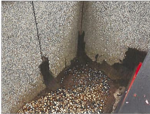
View of suspected prior repairs at the lap joints of the upturn flashing cap sheets of the BUR system.
