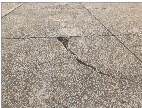
View of a linear crack within the concrete surface of the transport truck parking area at the south portion of the Site.
