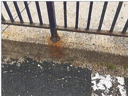
View of corrosion noted at the metal railing at the walkway adjacent to the southwest corner of the Site Building and at the patio area adjacent to the north elevation of the Site Building.
