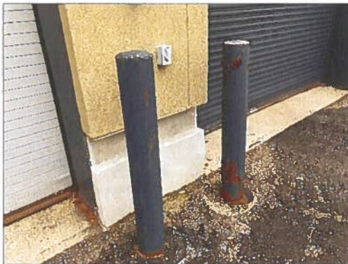
View of corrosion at steel bollards adjacent to the west elevation of the Site Building.
