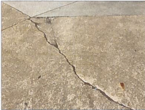
View of a linear cracking in a concrete walkway.
