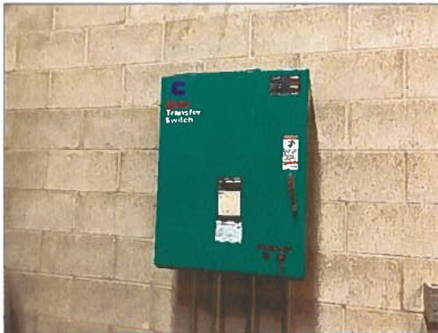
View of the automatic transfer switch serving the Site Building.
