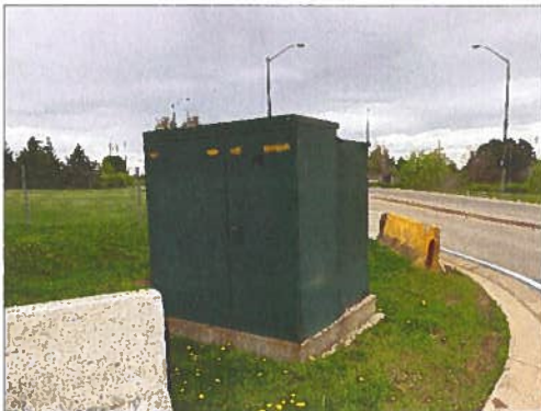
View of the pad-mounted transformer serving the Site.
