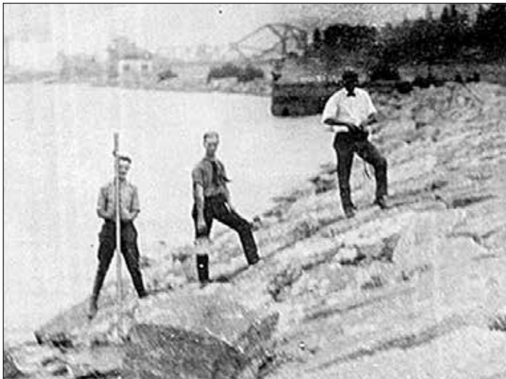
Surveyors ensure the bridge will be built in the right location.
